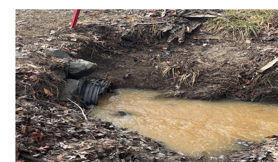
Current culvert inlet
