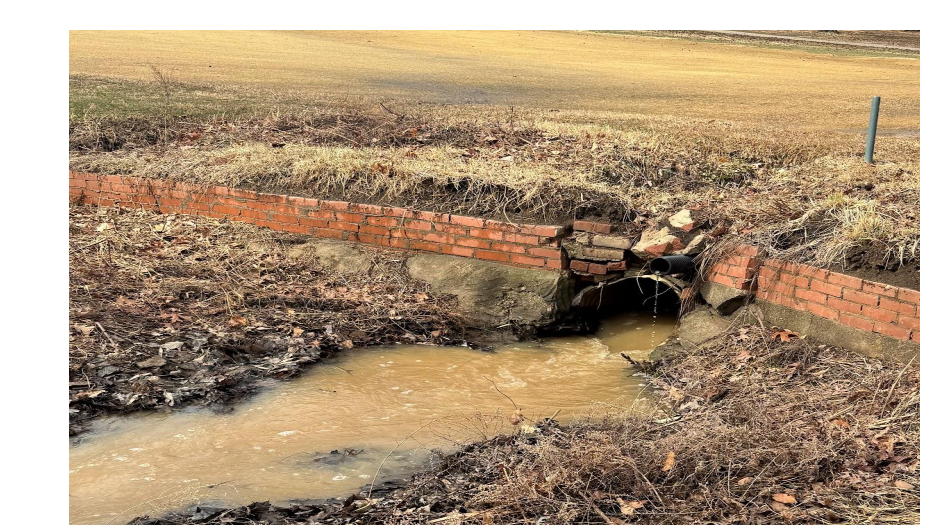
Current culvert outlet
