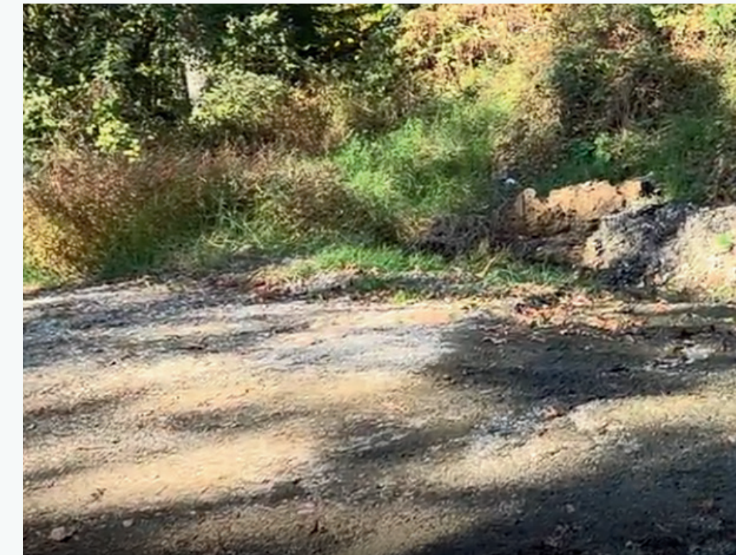
Figure 3: Current Washing Area is a Dirt Patch with Severe Erosion
