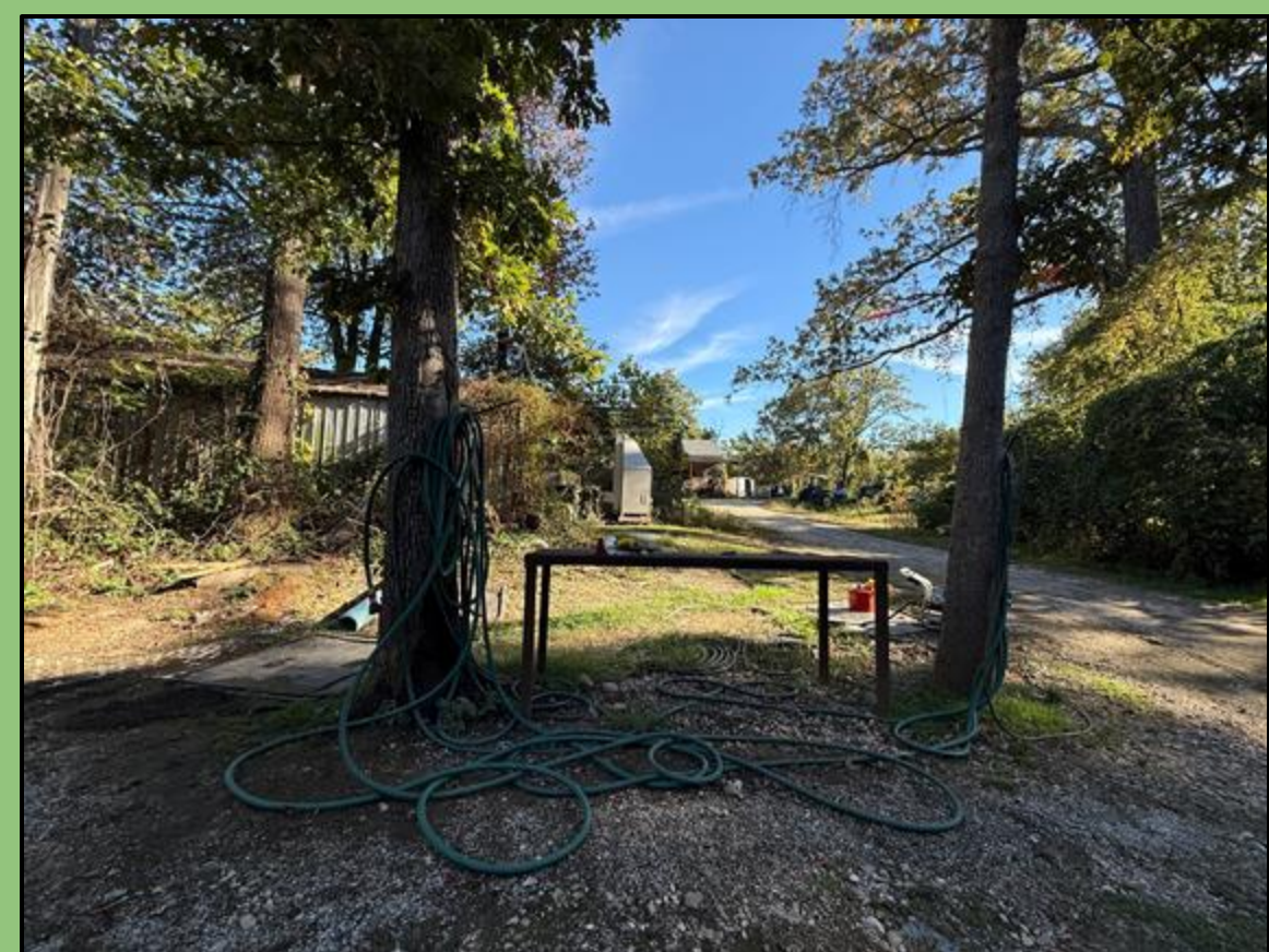
Figures 3-4: Current two wash stations on project site. Left image is for pressurized water washes used to clean 10-12 machines daily. Hoses are improperly stored and the surrounding area has become eroded due to runoff. Right image is for chemical washes next to the chemical storage cabinet.
