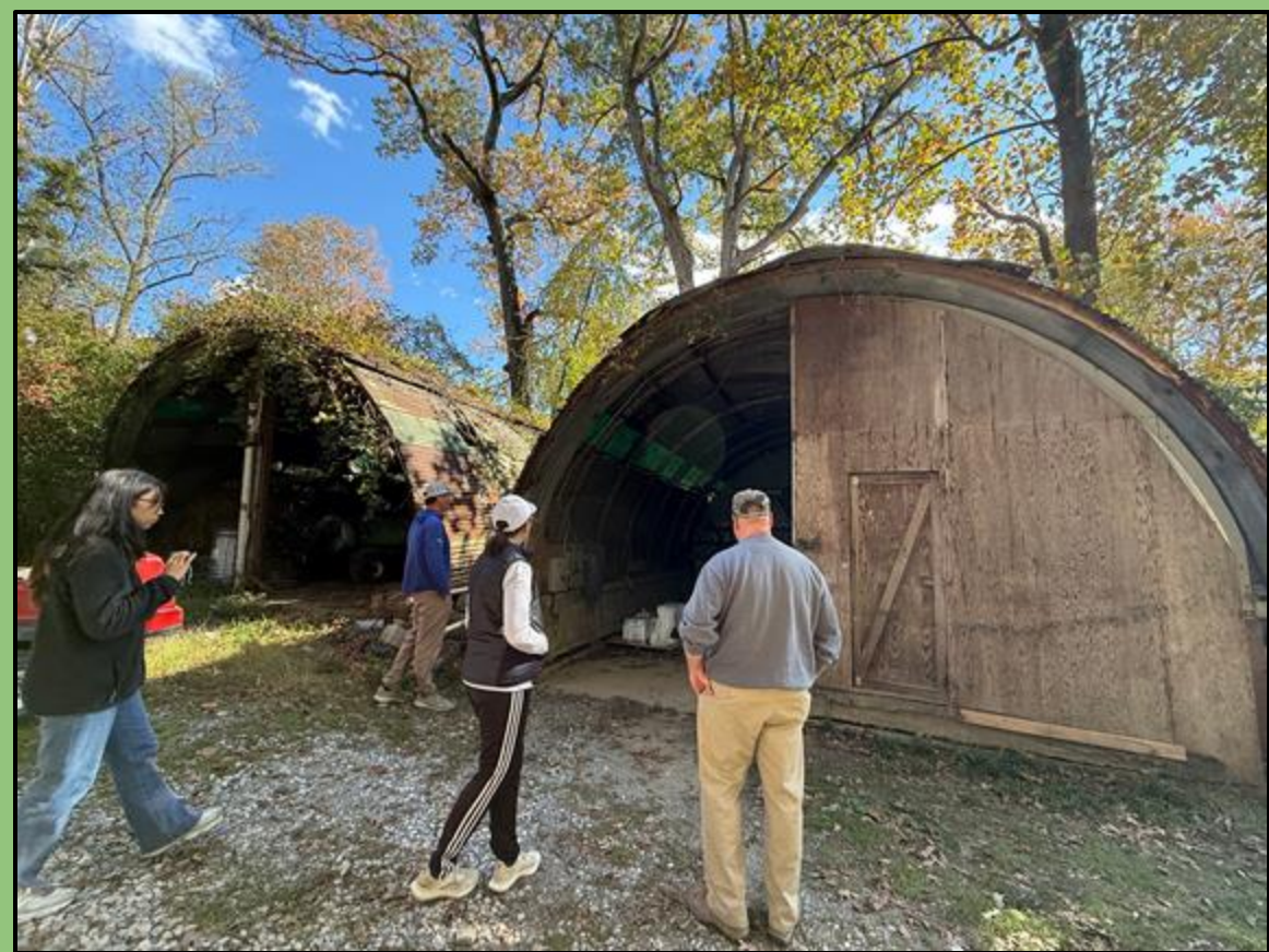
Figures 1-2: Current storage areas with deteriorated or missing structural wood, doors, and windows. Vehicles are scattered outside of the sheds due to the lack of storage space.
