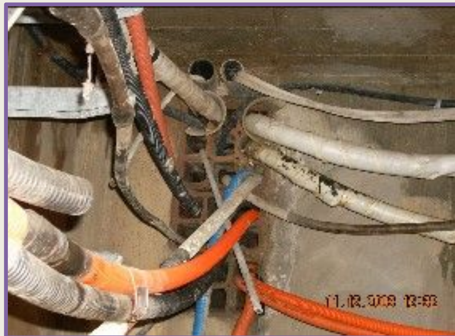
Original Condition of Baltimore City Conduit Section
